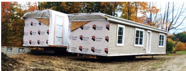
Figure 23. The Typical Double-Wide Mobile Home, Post-Delivery and Pre-Installation in Starksboro, VT
